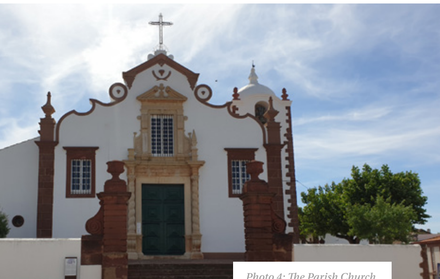
Photo 4: The Parish Church.
